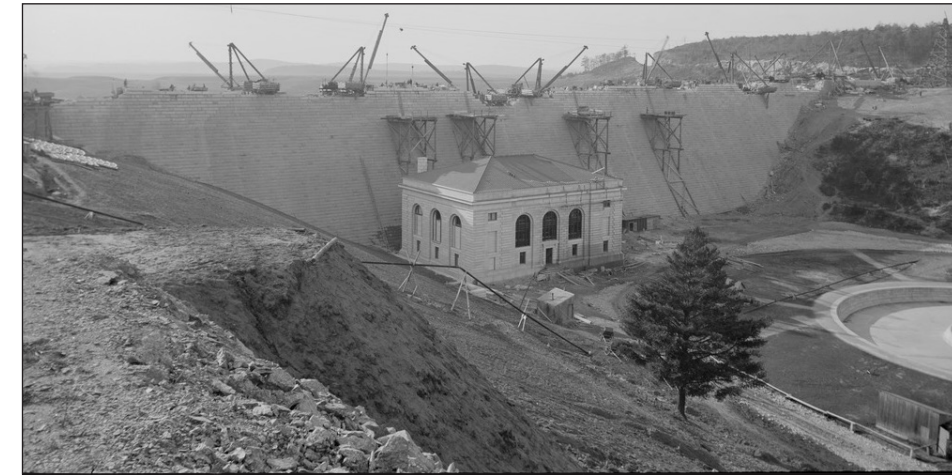
The Wachusett Reservoir, opposite page, was the largest man-made reservoir when it was constructed in the 1890s, left, by damming the Nashua River in the Worcester County town of Clinton, 35 miles west of Boston.
