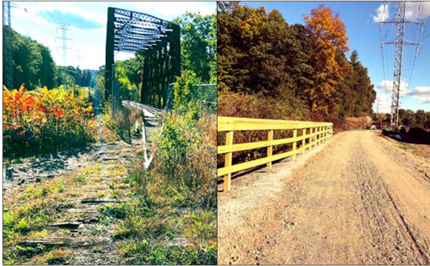
Left: 1896 trestle bridge over the Fitchburg Line tracks and unimproved future trail, photographed from the Waltham side. Right: Waltham segment 3, an unpaved path between Fitchburg Line and Jones Road.
