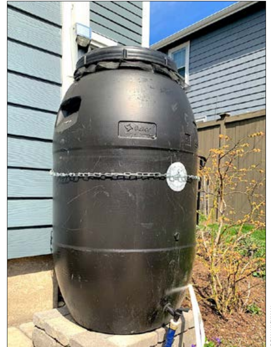
Rain barrel purchased several years ago with downspout diverter.
